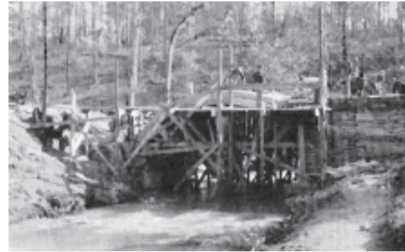
Construction of the arched bridge at Chewacla.
