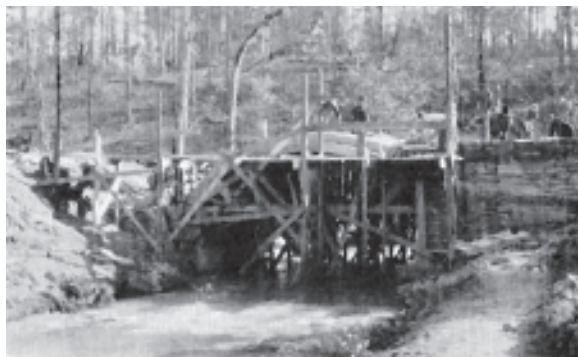
Construction of the arched bridge at Chewacla.
