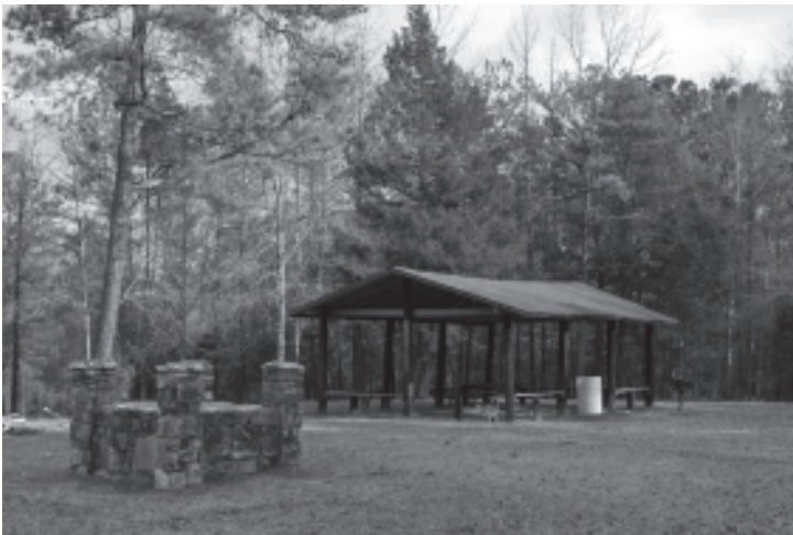
The CCC Camp pavilion near Chewacla State Park
