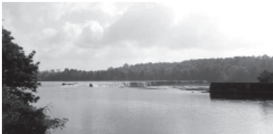
Langdale Dam, on the Chattahoochee River between Valley, Alabama and Georgia, was built about 1908.
