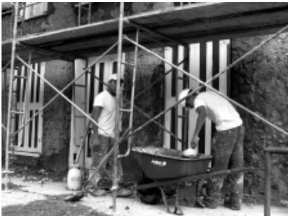
Workers from Simpson Plastering Co. remove and replace the exterior stucco on the Trade Center. The restoration should help preserve the building for another 164 years.
