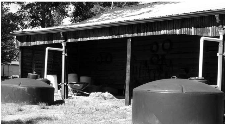
Two huge rainbarrel cisterns on the west side of the McLain Building collect runoff from the building to water the new Grandma's Flower Garden and the McLain Garden. A third cistern is hidden underneath the Millstone Fountain. Together, the three cisterns can store almost 4000 gallons of rainwater.
