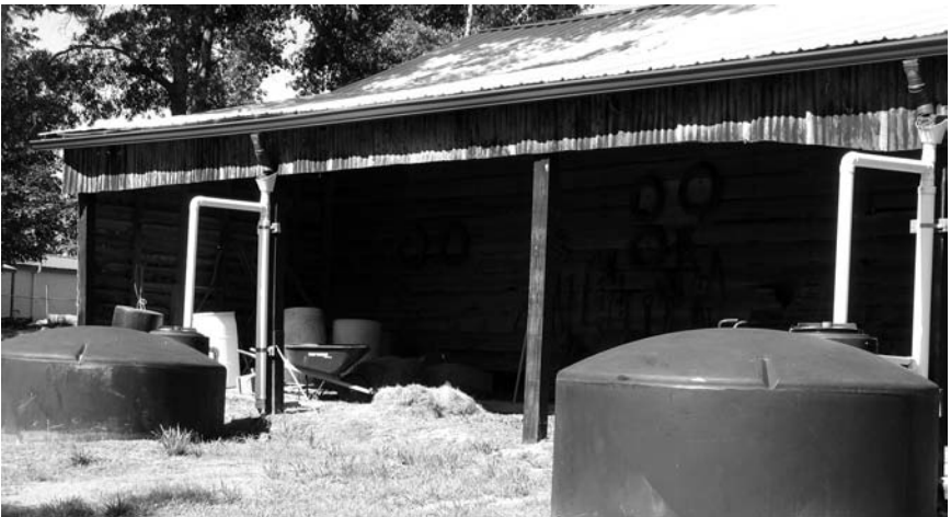
Two huge rainbarrel cisterns on the west side of the McLain Building collect runoff from the building to water the new Grandma’s Flower Garden and the McLain Garden. A third cistern is hidden underneath the Millstone Fountain. Together, the three cisterns can store almost 4000 gallons of rainwater.
